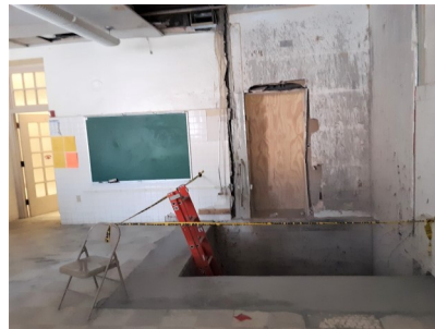
New Elevator Shaft
